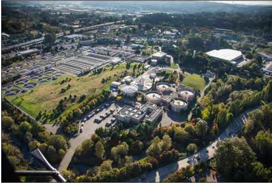
Figure 15: Low Solids (POTW) AD Plant, Renton, WA
