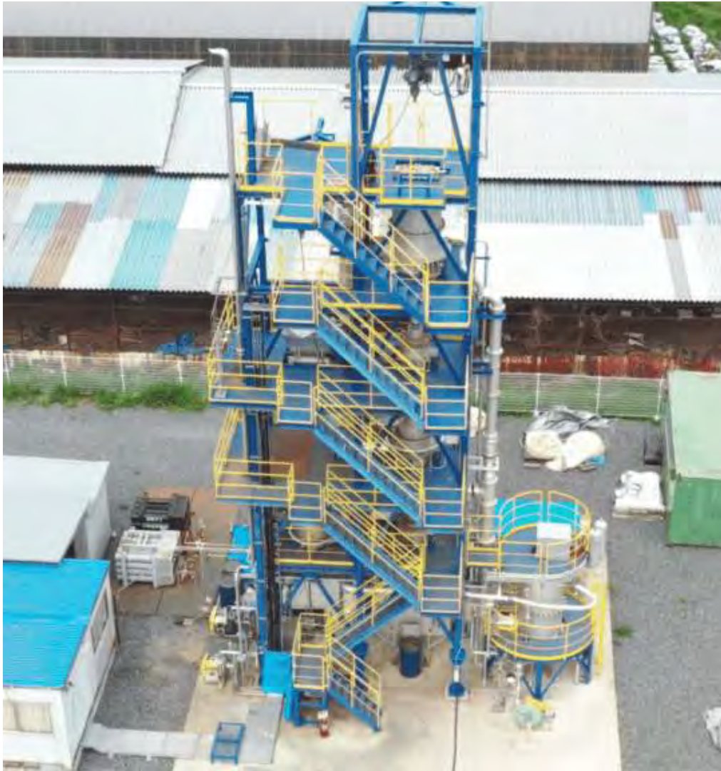
Figure 7: Ways2H Pyrolysis Facility Kern County, CA
