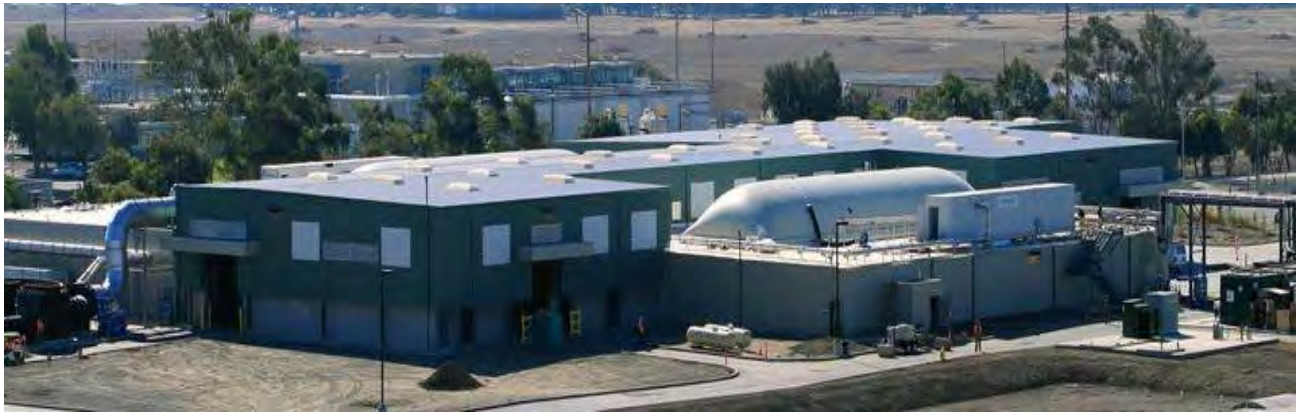
Figure 19: Zero Waste Energy Development Co. AD Plant, San Jose, CA
