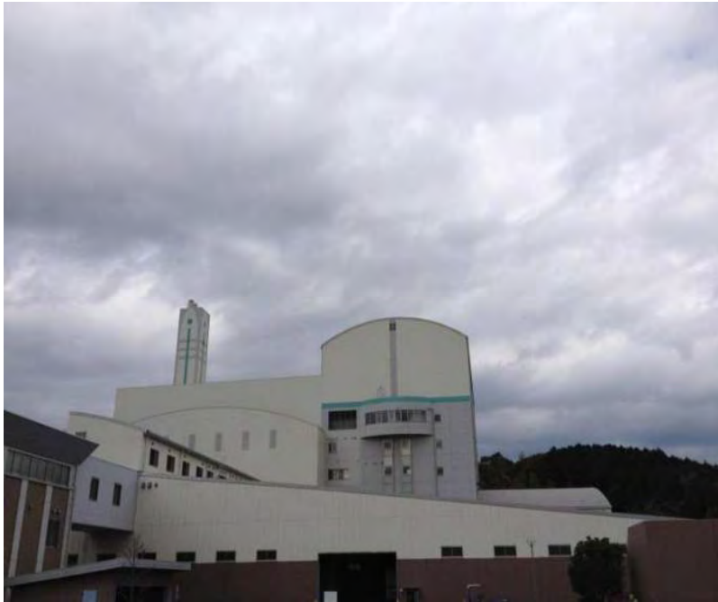
Figure 3: Homan Gasification Plant (Fukuoka, Japan)
