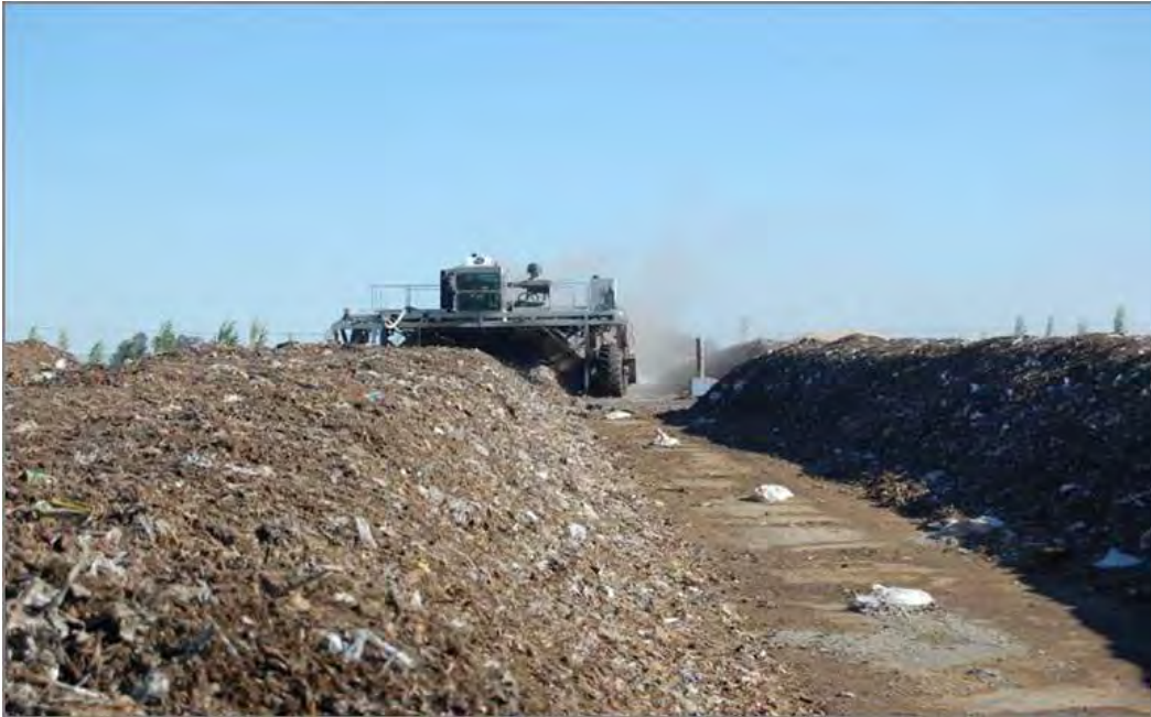
Figure 8: Example of a Windrow Aerobic Composting Facility
