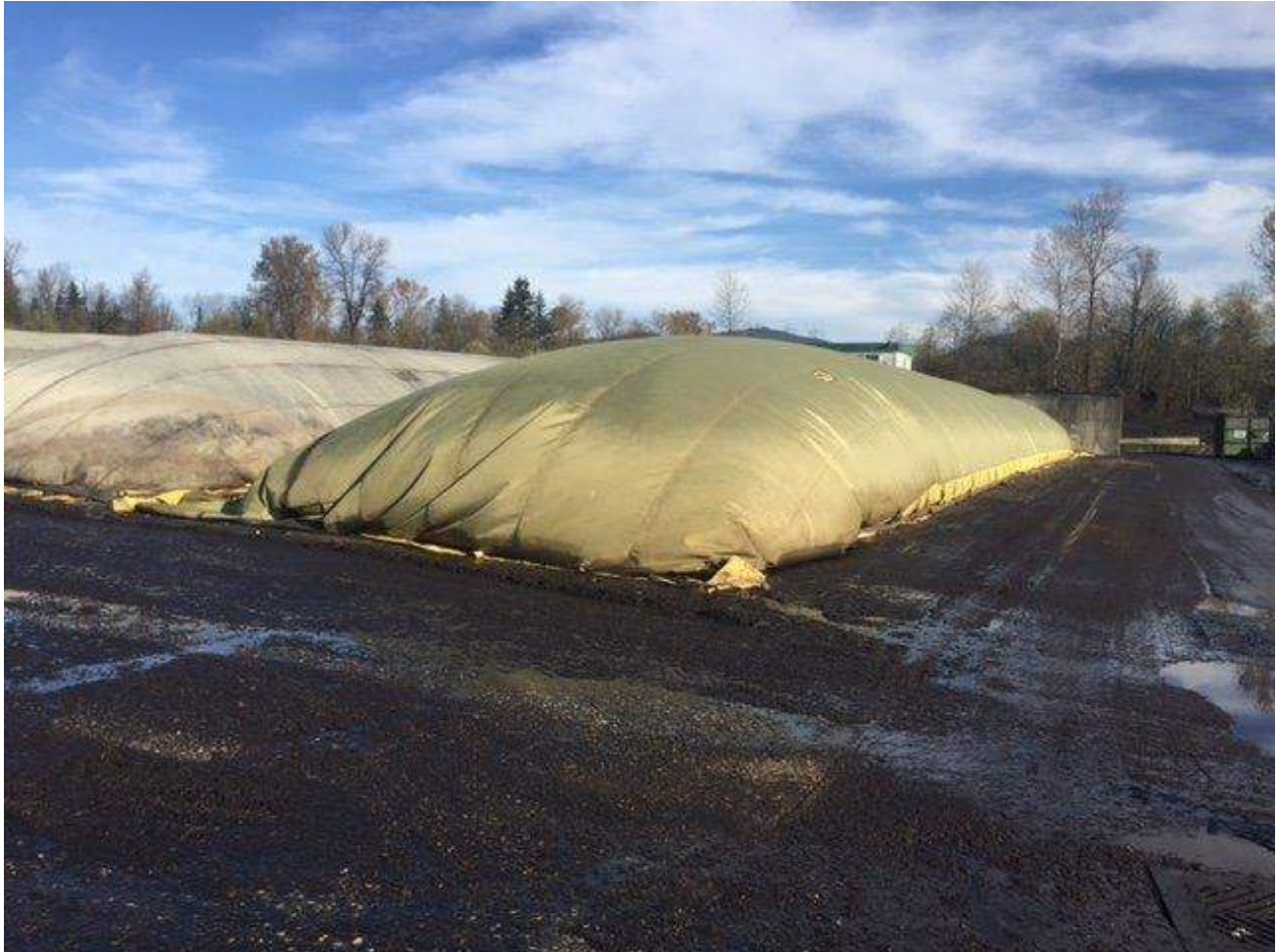
Figure 9: Example of a Fabric Covered Aerobic Static Composting Facility, Issaquah, WA
