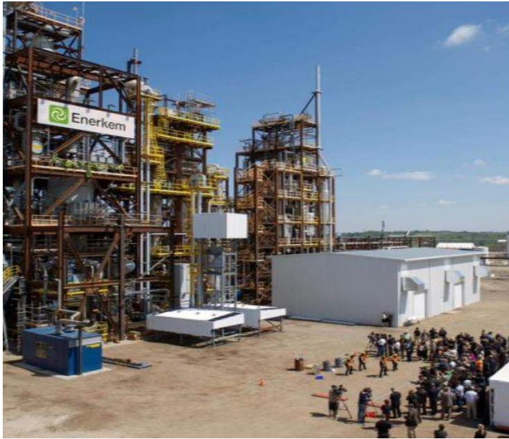
Figure 22: Enerkem Alberta Biofuels Facility, Edmonton, Alberta, Canada
