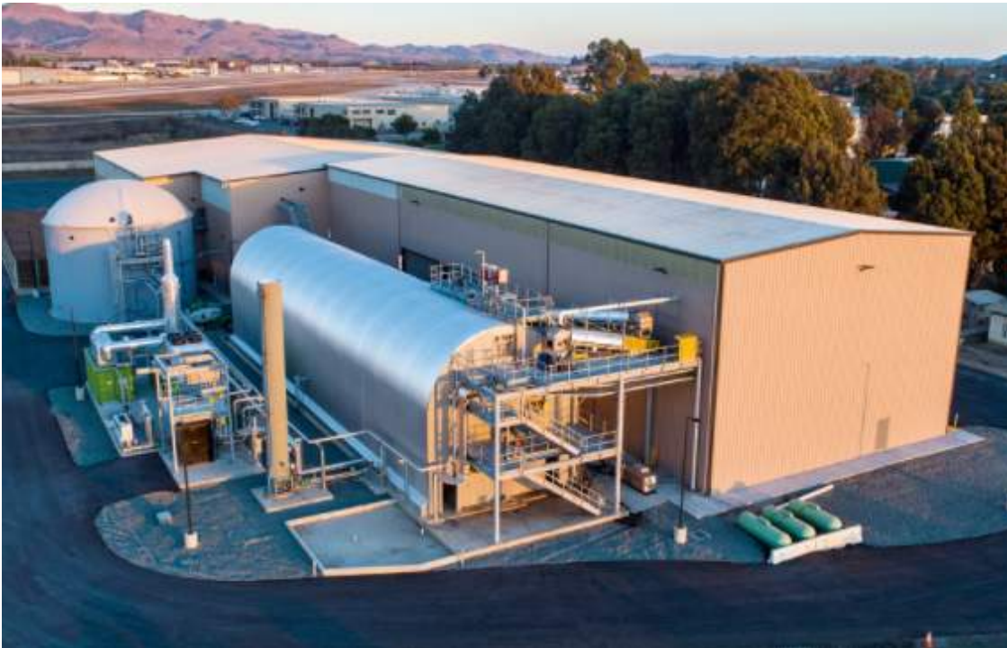
Figure 16: High Solids Horizontal AD Plant, San Luis Obispo, CA
