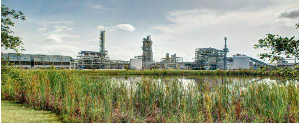
Figure 23: Indian River Biofuels Facility in Vero Beach, Florida
