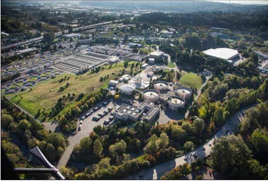
Figure 15: Low Solids (POTW) AD Plant, Renton, WA
